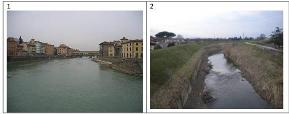
Figure A3. 54 Cases of bank-edge levées occurring for most of the reach. In this case, an <u>additional score of 6 or 12</u> (depending on the % of the reach length) is added.
