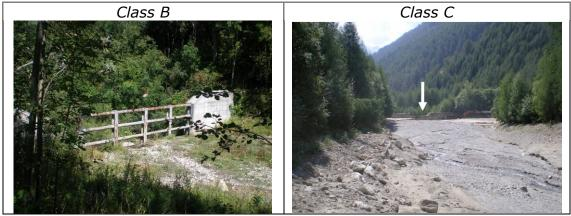
Figure A3.2 (continued) Longitudinal continuity in sediment and wood flux. Class A: absence of discontinuities. Class B: up on the right, filled consolidation check dams; low on the left, open check dam. Class C: a check dam (arrow) with total interception represents a complete alteration of longitudinal continuity in the reach downstream from the check dam.
