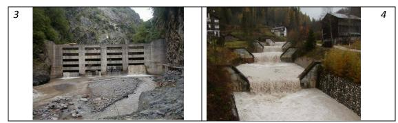
Figure A3. 39 Transversal structures of alteration of sediment discharges in mountain areas. (1) Dam; (2) retention check dam; (3) open check dam; (4) sequence of stepped consolidation check dams.
